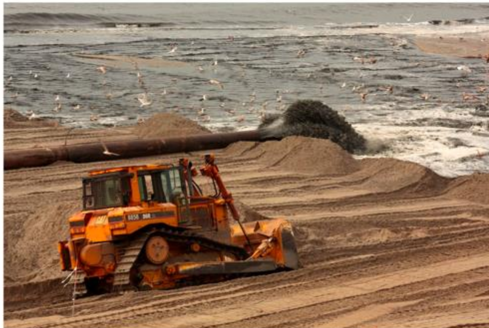
A beach replenishment project underway at Rockaway Beach in New York in 2014, following Hurricane Sandy. (Carolyn Cole/Los Angeles Times via Getty Images)
