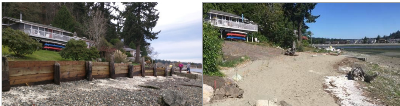
A property on the Puget Sound before and after removal of the bulkhead. Photos from: Shore Friendly program, Puget Sound Institute
